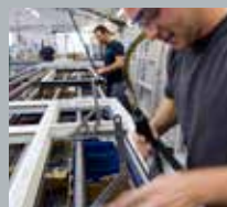
FABRICATE NEW WINDOWS
